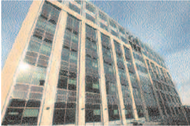
Solar panels mounted on the Brewery Block buildings in Portland GERDING/EDLEN
