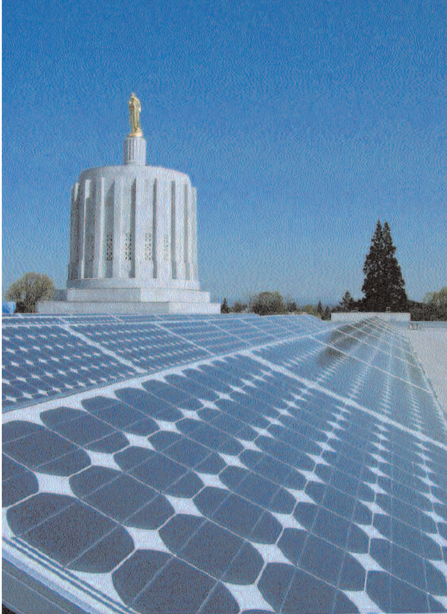
The solar array on Oregon's State Capitol building in Salem is used to light its Pioneer statue OREGON DEPARTMENT OF ENERGY
