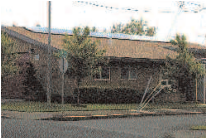
Solar on the roof of a fire station in Portland
